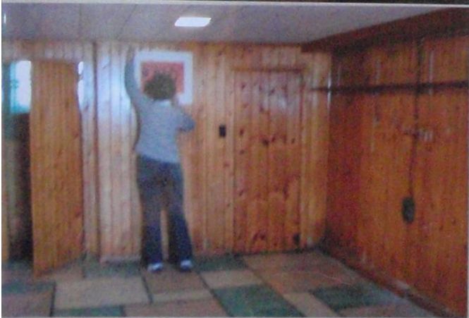
Down to the bare walls!
